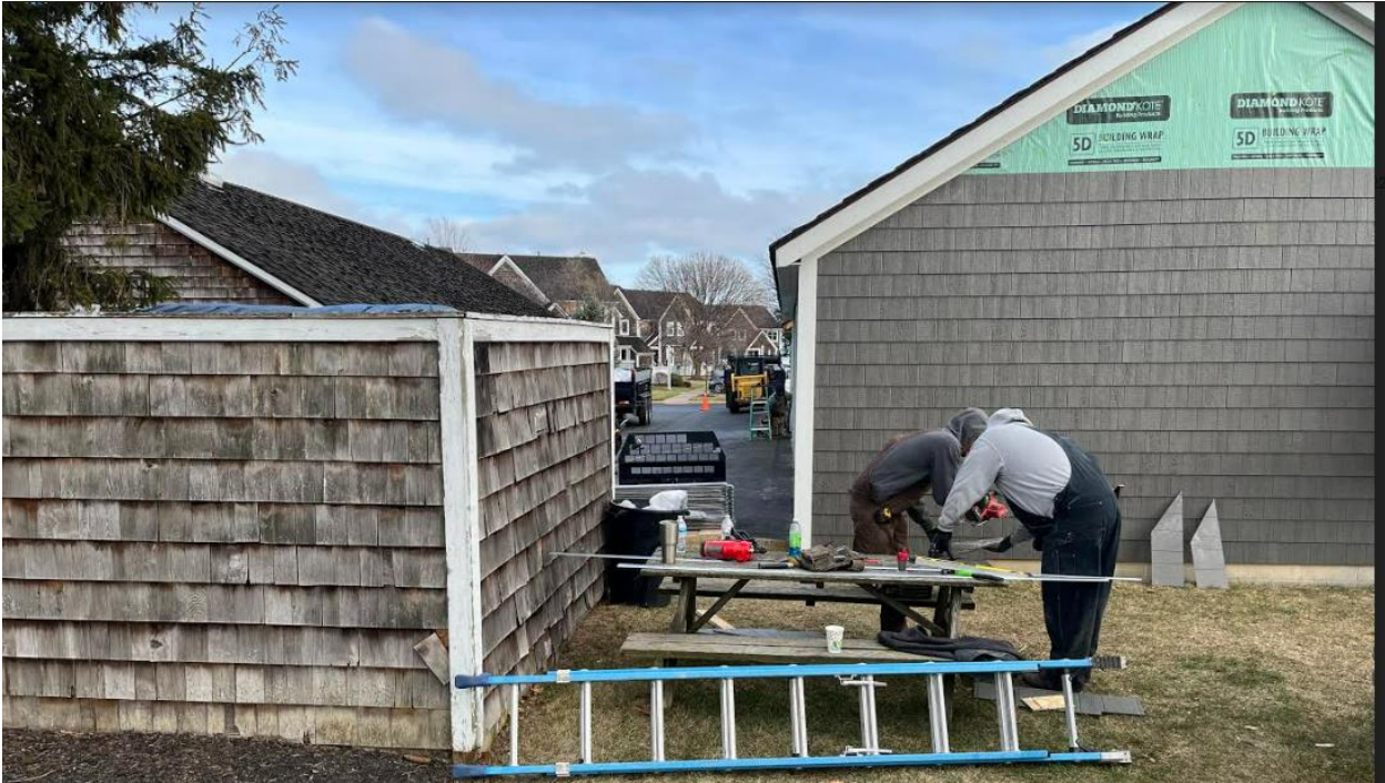
Contrast pic between new siding and dumpster enclosure
