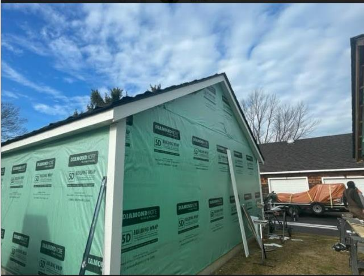
Garage trim going up
