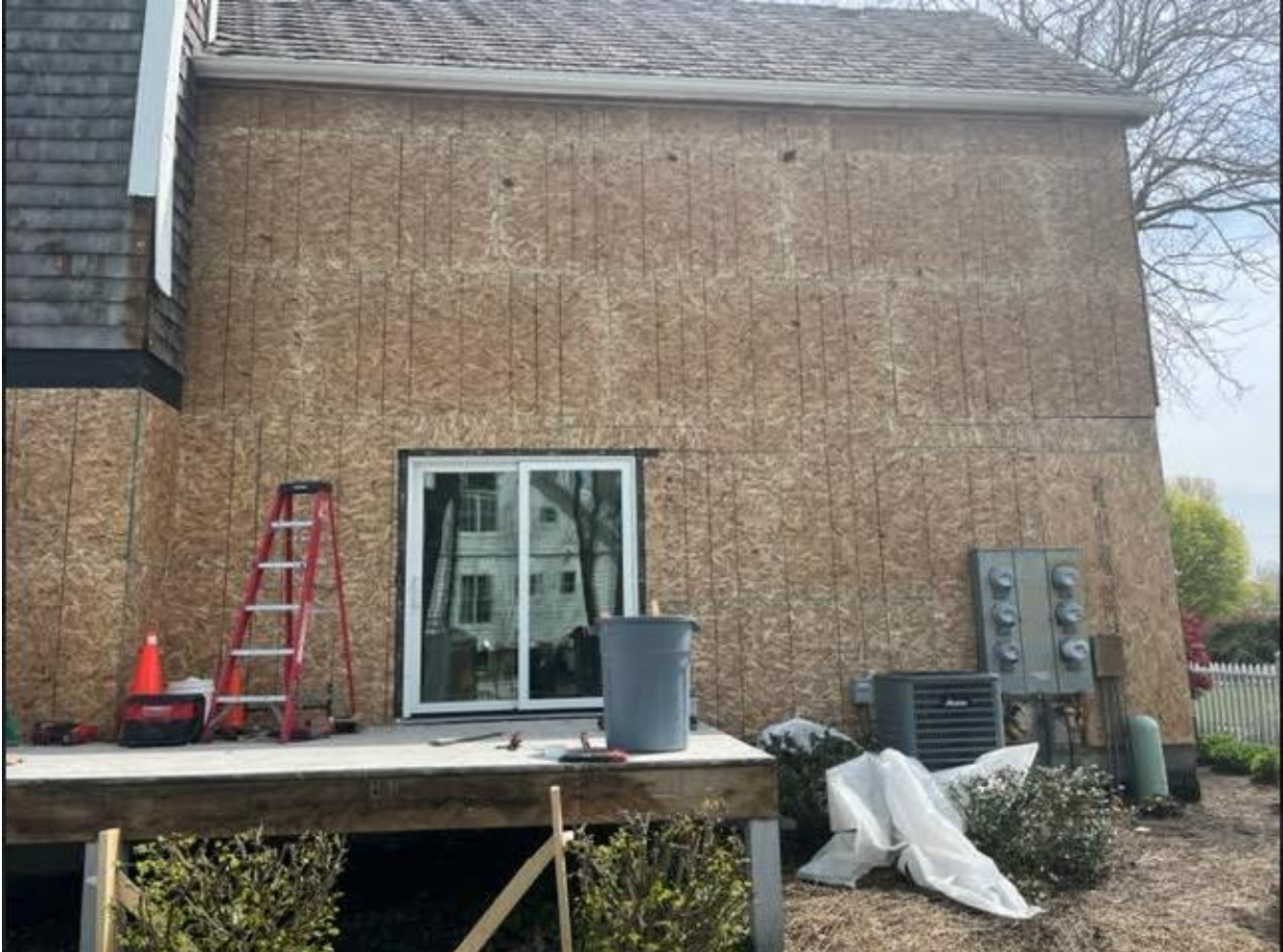
OSB installation has begun on building 1.
