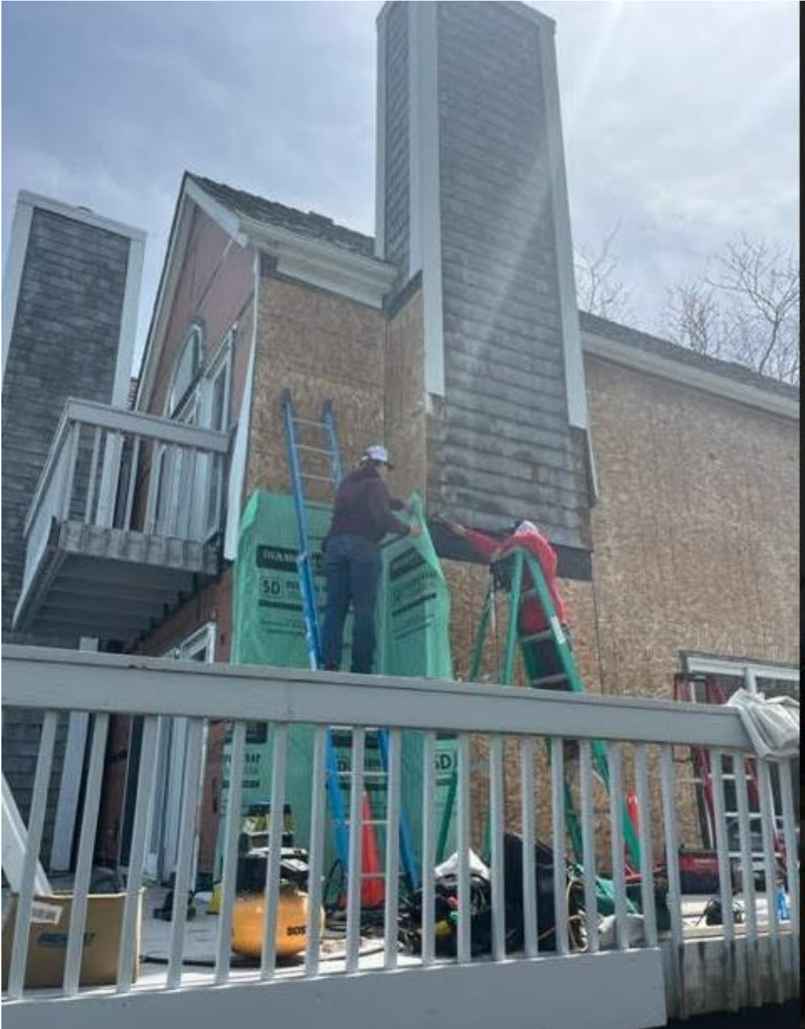
Vapor barrier being installed on building 1.
