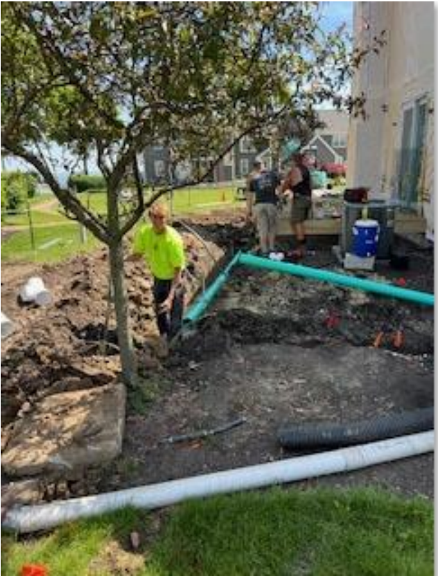
Tying in Bldg 4 and 5
