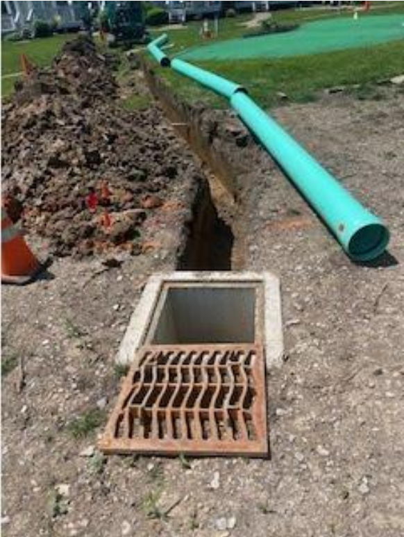
Drain to Catch Basin
