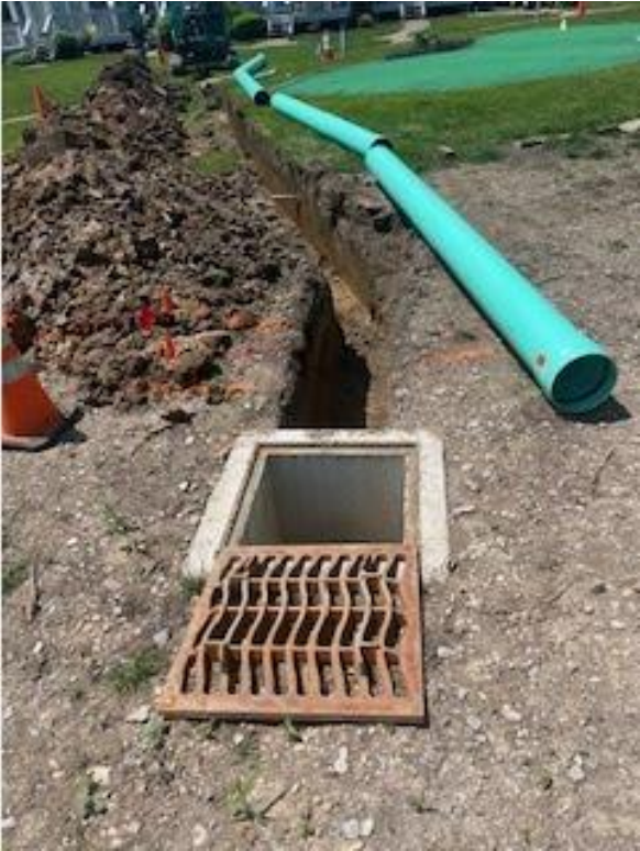
Drain to Catch Basin
