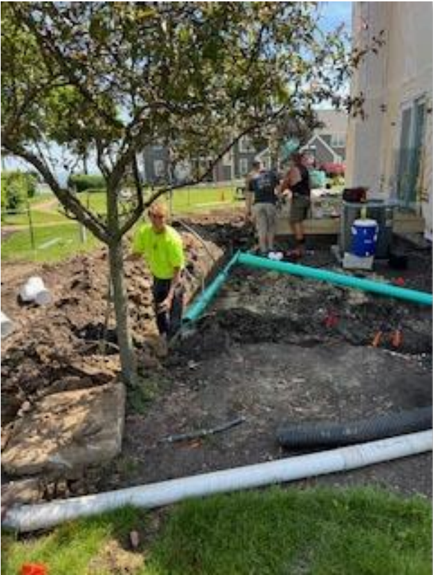
Tying in Bldg 4 and 5
